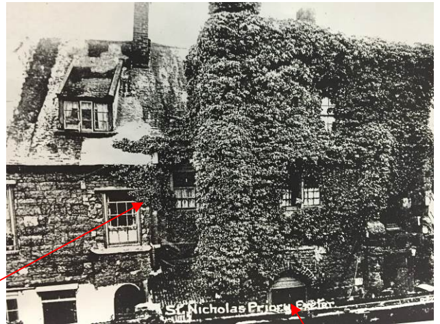
Ground floor tower room window was a door
