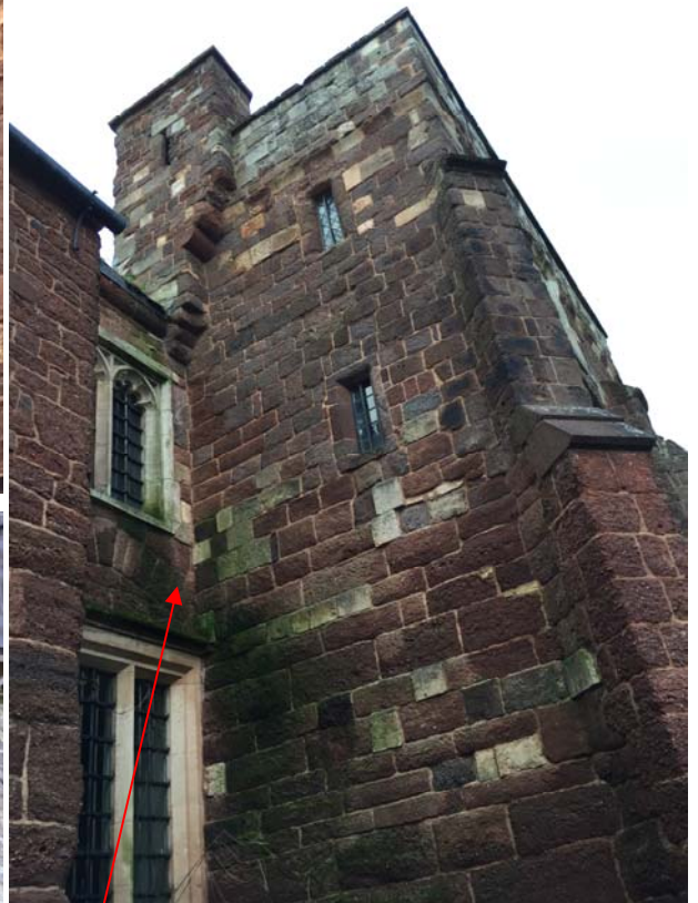
Because this gutter is blocked, the stone below is saturated and stained.
