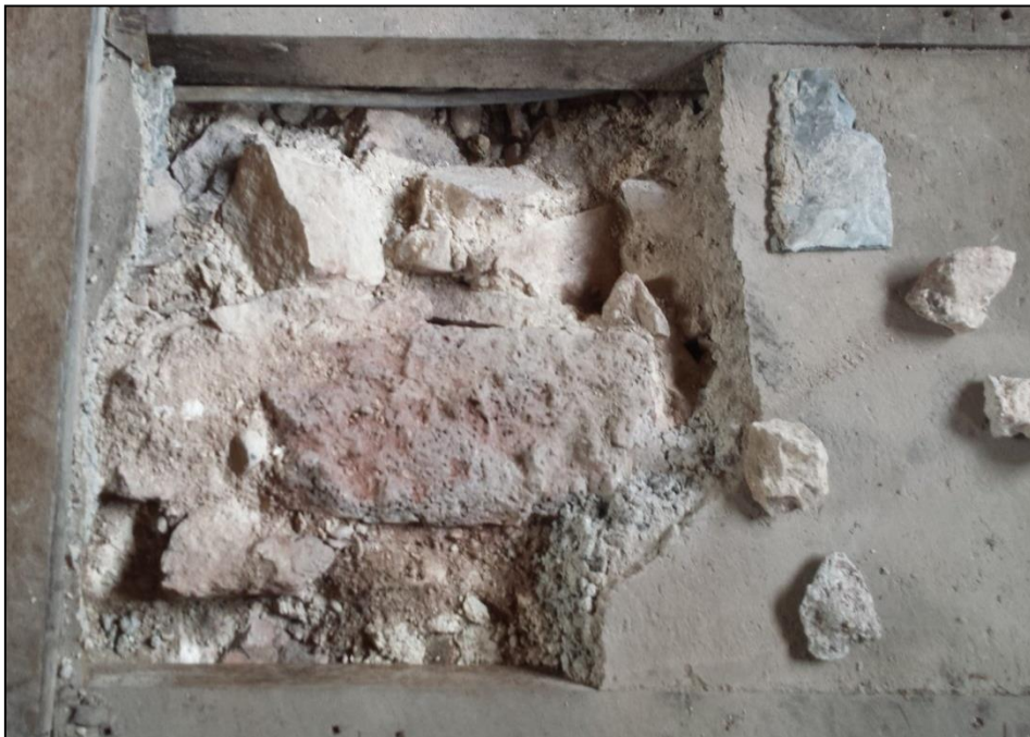
Image of the trial hole one following excavation and vacuuming.
