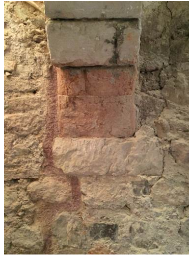
Arch not central to corbel with newer stones above first two courses.
